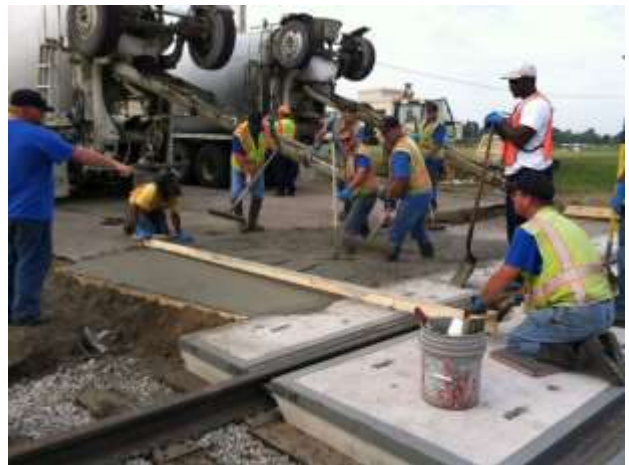
DPW CREW REPAIRS N. WEST ST. RAILROAD CROSSING
