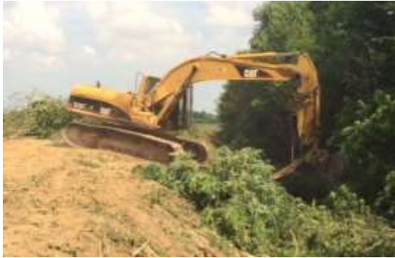
GREENBRIER DITCH CLEAN-OUT
