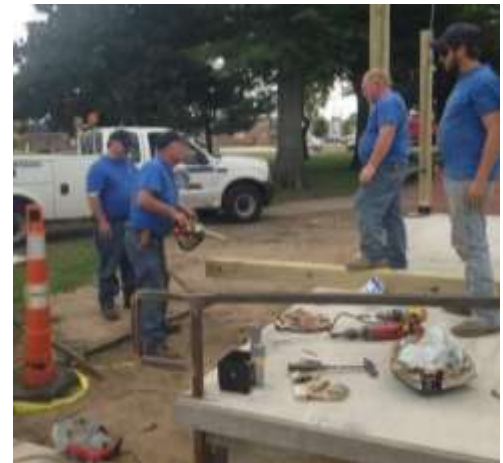
LEGION PARK BAND STAND UNDER CONSTRUCTION
